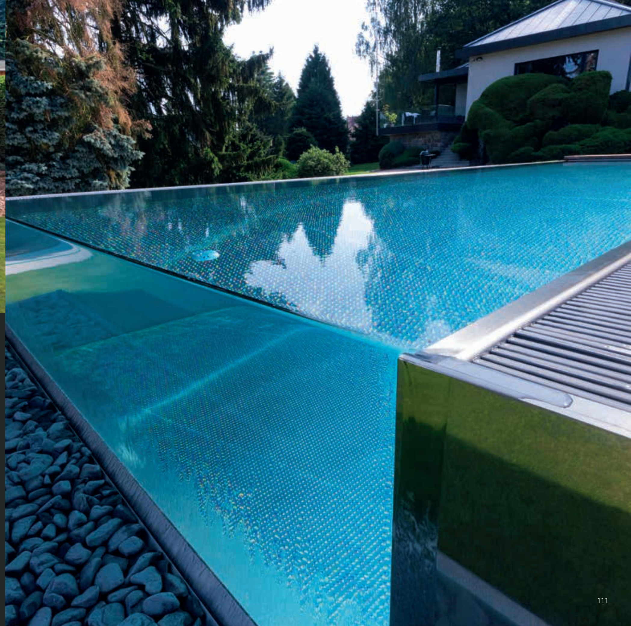
Overflow above the glass partition and gutter concealed beneath rounded stones
